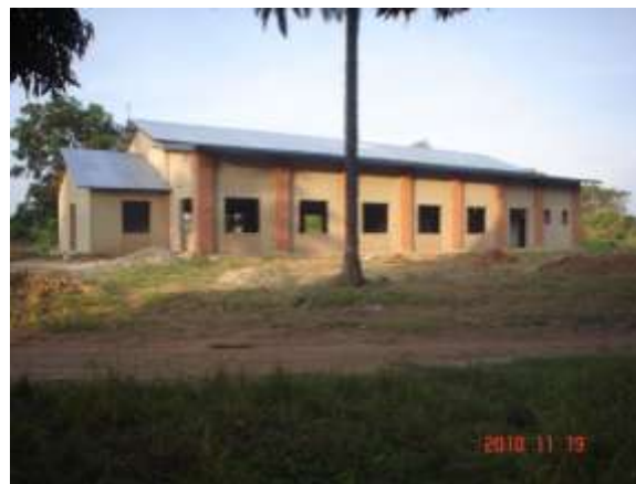
Cathedral Construction in progress
